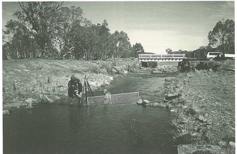
Penstock Lagoon project... the dog helped a lot
