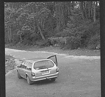
Resurfaced roadway at Lake Echo Dam
